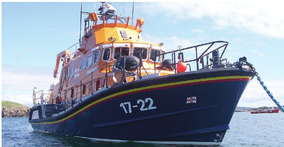
Plans have been submitted for a state-of-the-art RNLi lifeboat station on the Donegal island of Arranmore on the site of the current station on the NE side of the island. The original RNLi station was first established in 1883 with the present all weather station opened in 1997 by Daniel O'Donnell.
